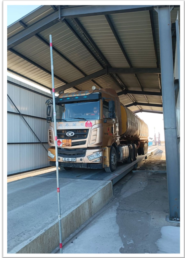
Tanker at Block XIX TA-1 Facility Weighbridge
