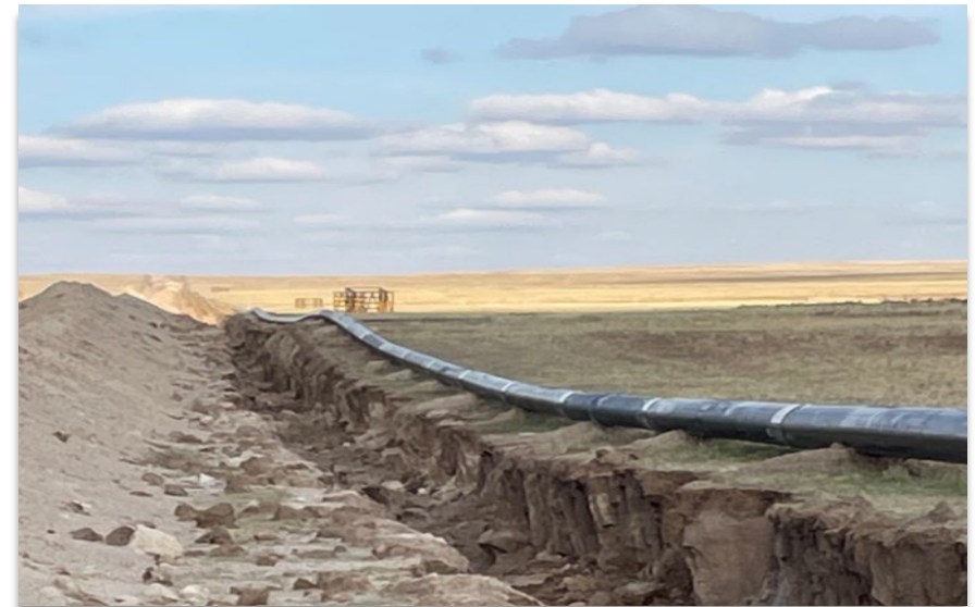
Picture of 20" pipeline installation en route to Block XX
